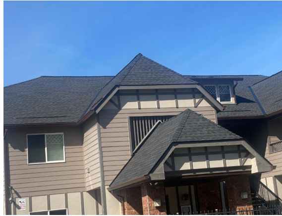
Roof-Composition-Asphalt-Phase 1
